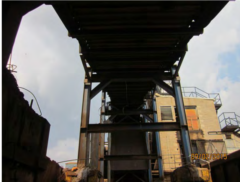
Structural cross supports in great condition
