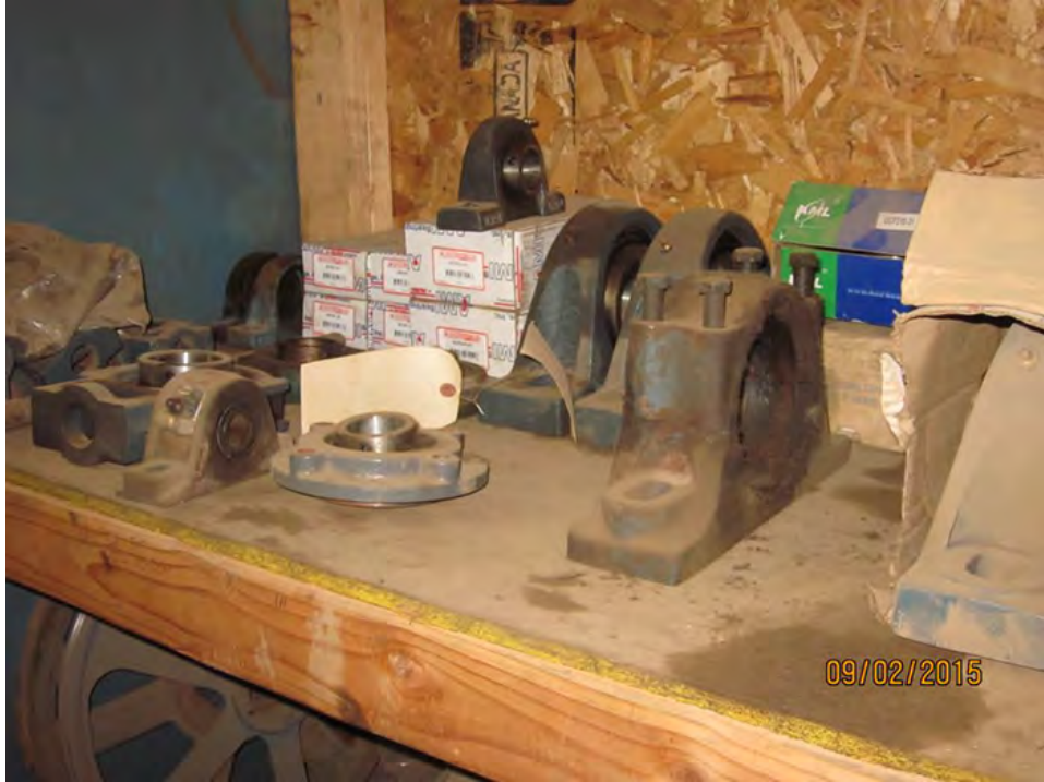
Spare conveyor bearings
