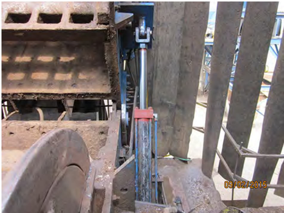
Base box walls in good condition
