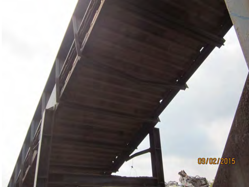
Structural frame work in good shape under the main frame
