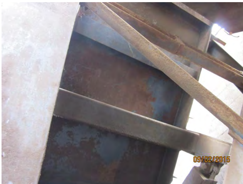
Bottom of chute fabrication in good solid welded condition
