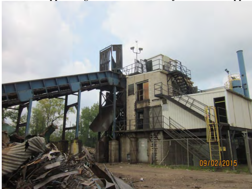
Main Structural Support in good condition. No major material trapped on belt
