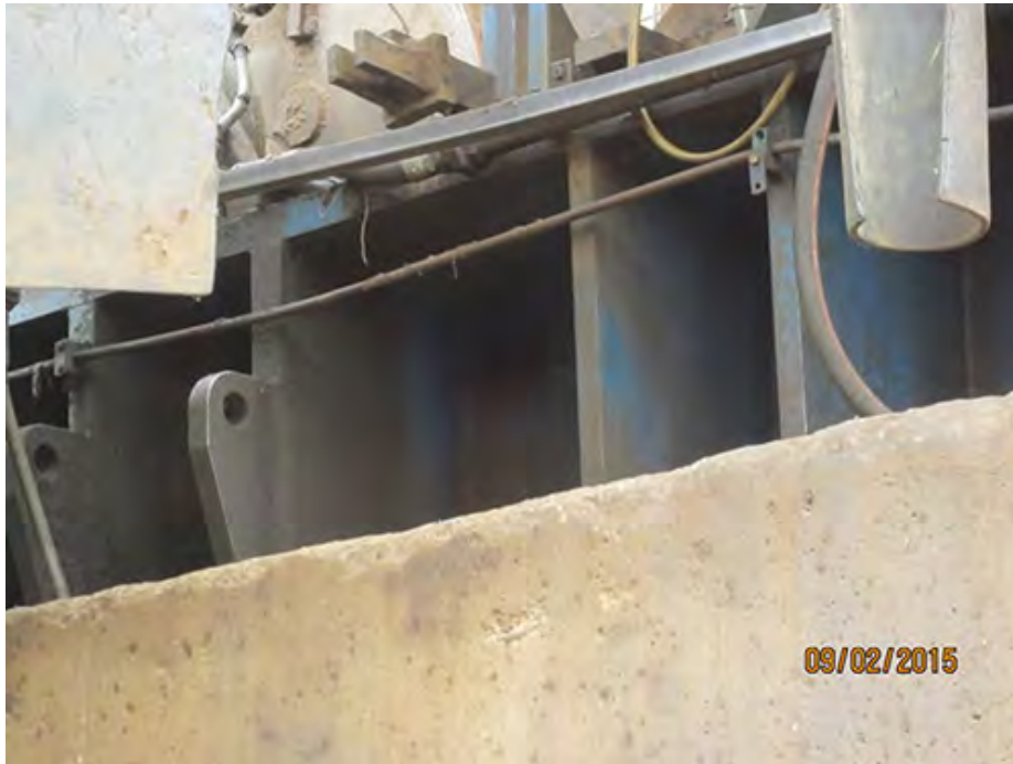
Base weld gussets no cracks evident in excellent condition
