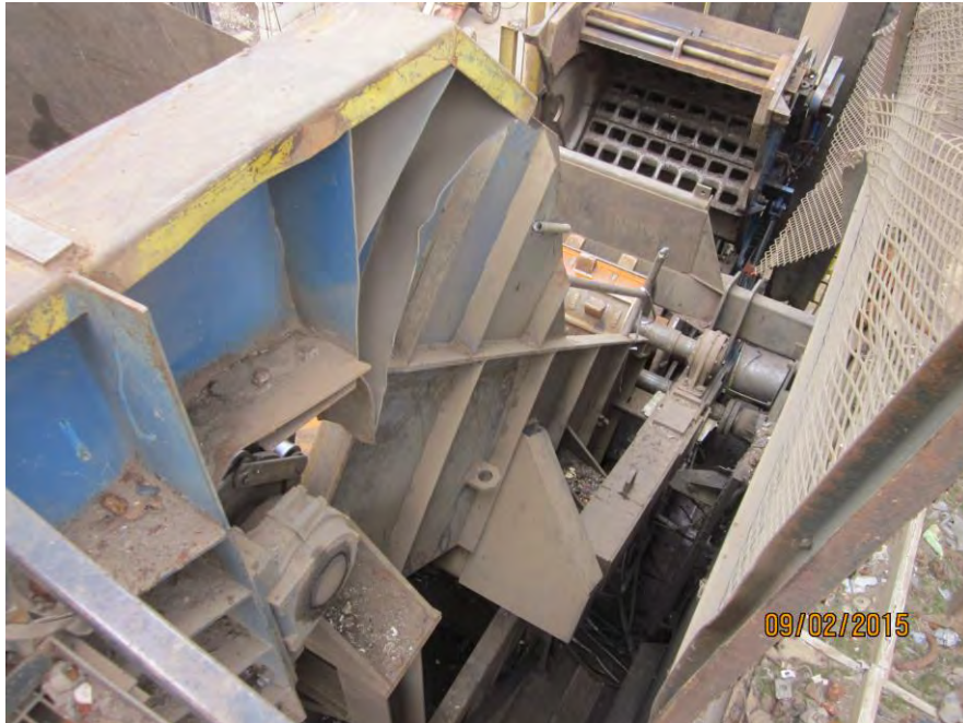
Outside walls of chute in excellent shape and straight
