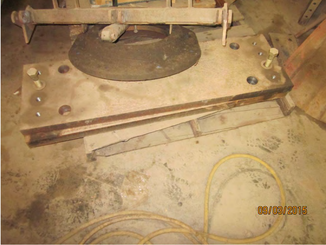
Bearing shim plates (replacements new)
